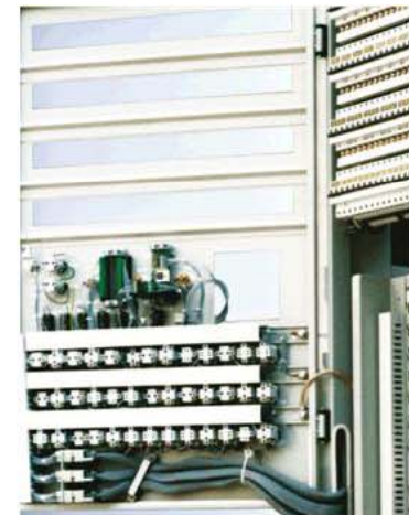
ELECTRO MECHANIC SYSTEMS
